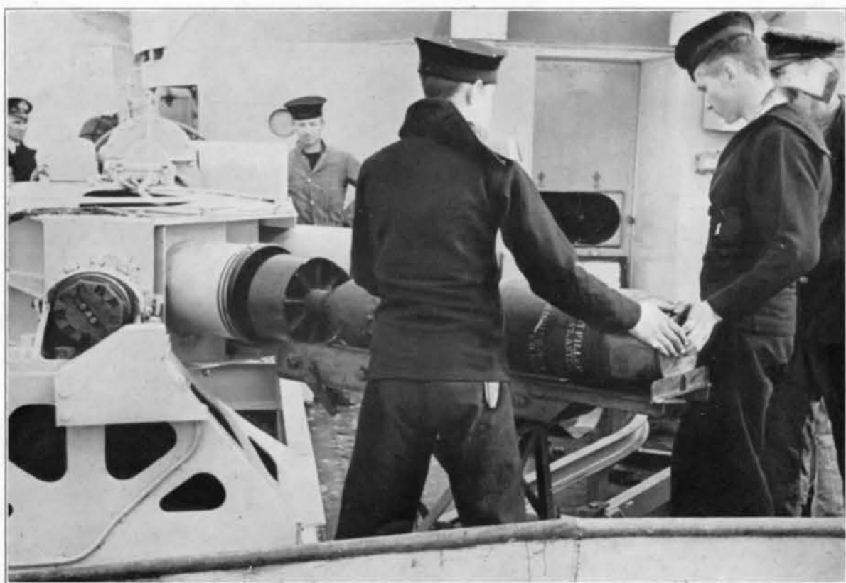
Mounting in Loading position. Showing method of loading.
